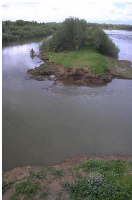
CLOSEUP OF THE LEVEE BREACH
