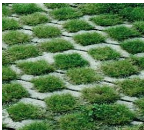
EXAMPLE OF PERMEABLE PAVEMENT
