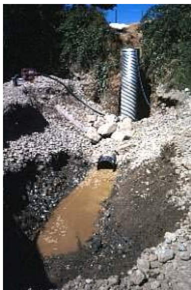
INFILTRATION GALLERY DURING CONSTRUCTION ON SUCKER CREEK, OR
