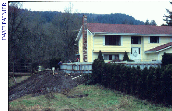
FLOOD WALL BEING ERECTED FOR PRIVATE LANDOWNER
