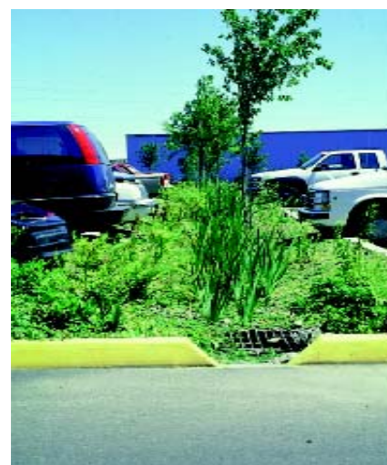
PARKING LOT SWALE FOR GROUNDWATER REPLENISHMENT AND CAPTURING RUNOFF
