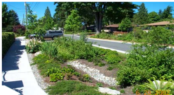
STREET SWALE IN SEATTLE
